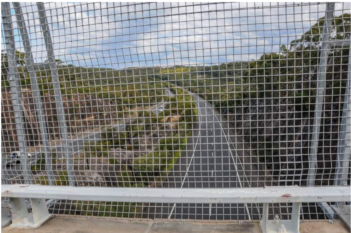
Cawley's Road bridge view looking south from the bridge showing the great division of the natural landscape and obstacle to wildlife movement presented by the F6 freeway.
