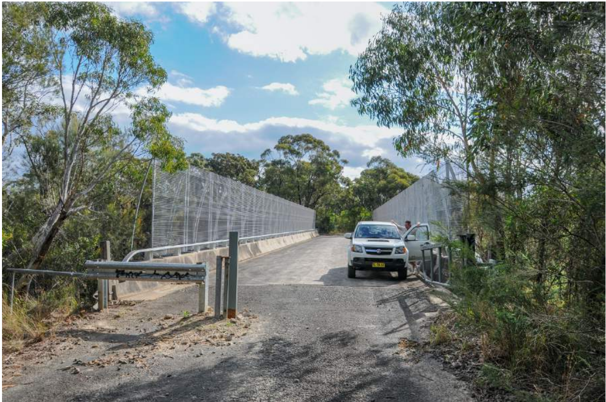
Cawley's road bridge viewed from the east side
